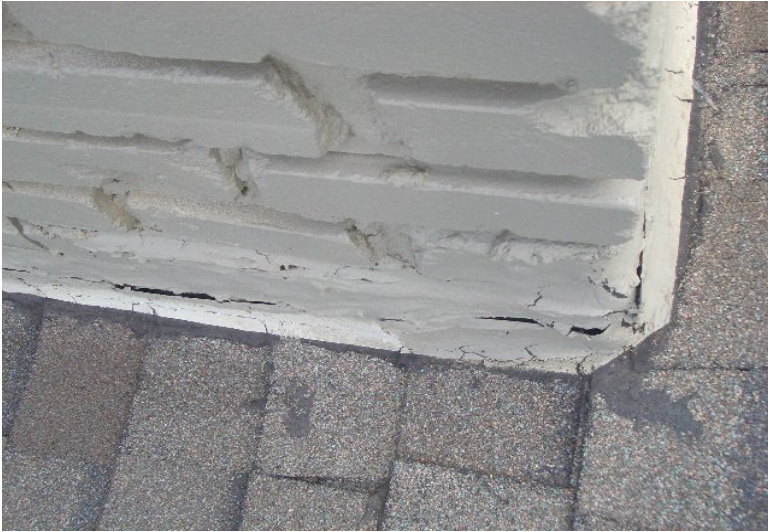
309. Open Seams noted at aged vent collars
