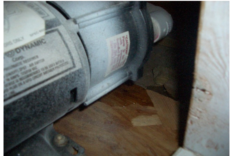
402. Leakage Noted At Whirlpool
