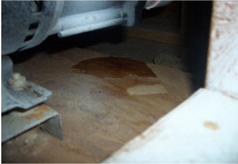
403. Leakage noted at drains/connections
