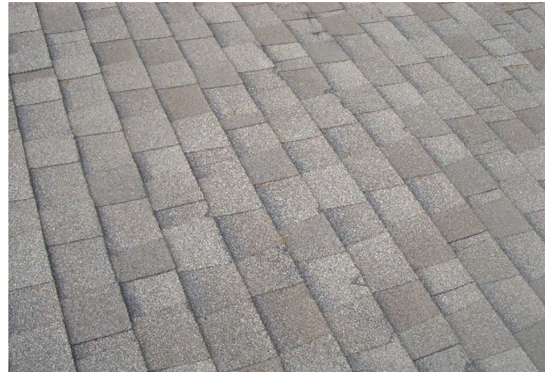
307. Prior Limb Contact Noted With Roofing Material
