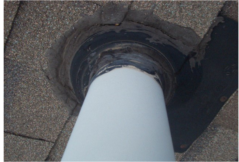
312. Surface Damage noted to roofing material
