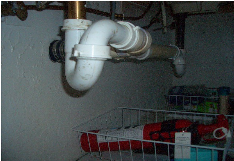
403. Leakage noted at drains/connections
