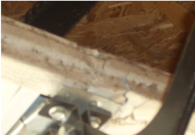
215. Damaged Garage Door Panels
