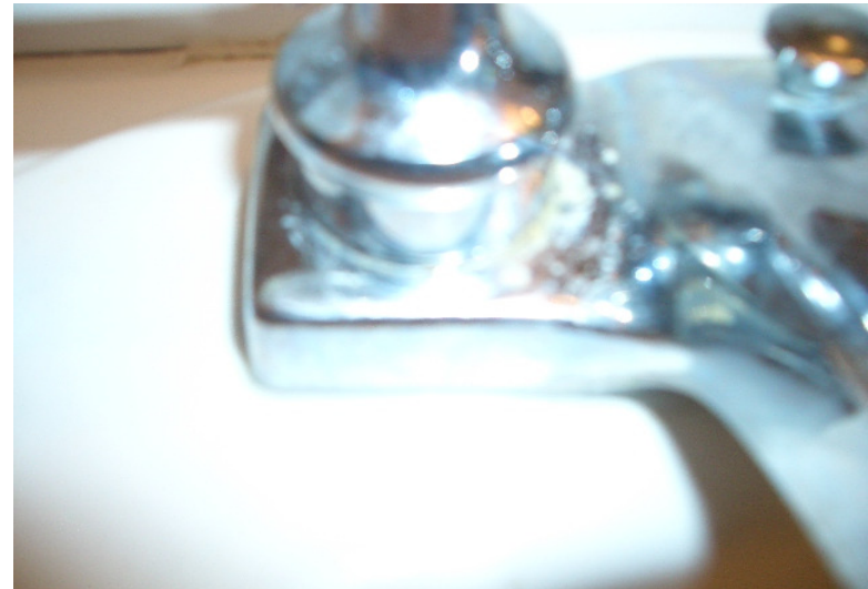
405. Leakage Noted At Base/Handle Area Of Faucet
