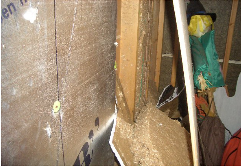
331. Dislodged / Missing Insulation Noted
