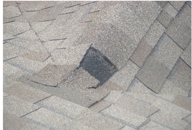
312. Surface Damage noted to roofing material
