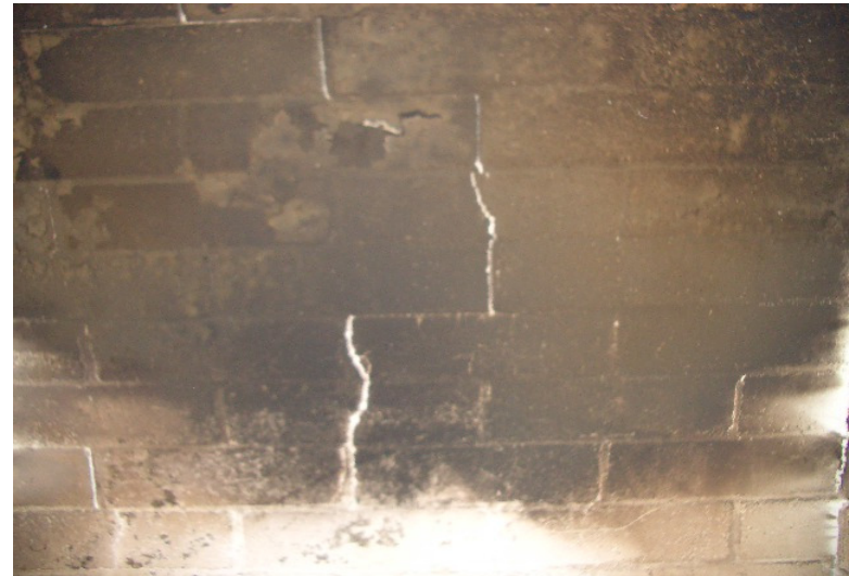
826. Defective Firebrick / Cracked Refractory Panel
