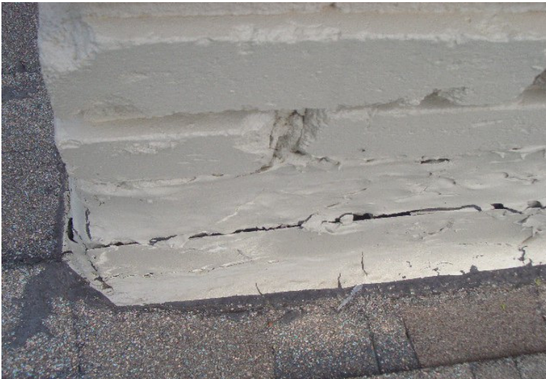
309. Open Seams noted at aged vent collars
