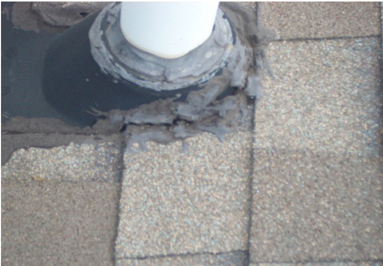
309. Open Seams noted at aged vent collars
