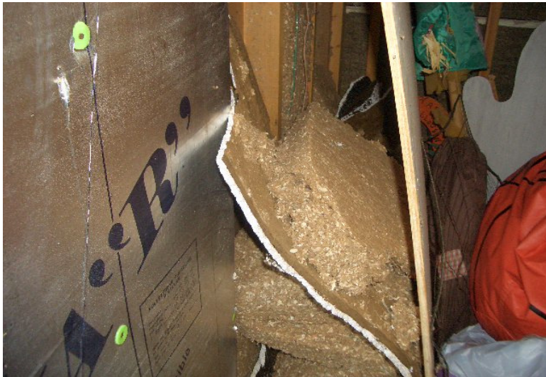
331. Dislodged / Missing Insulation Noted
