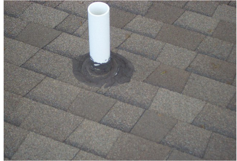
309. Open Seams noted at aged vent collars
